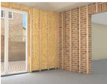
The interior has services added and is battened ready for internal finish.
