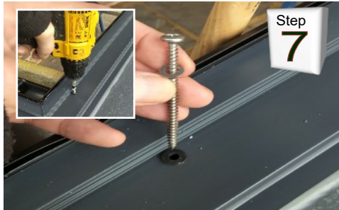
Insert 80mm screws into rubber fixing points on frame.
