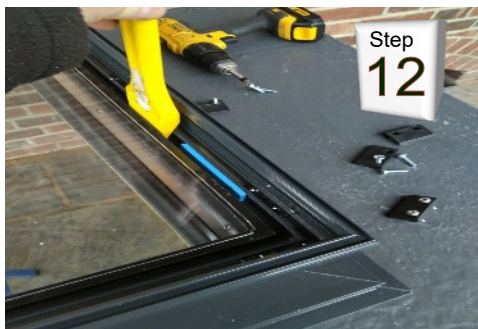
Pack glass unit evenly with glazing packers.
