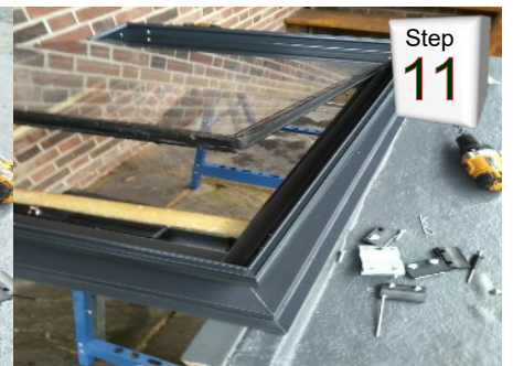
Glaze glass unit up the correct way, see glass label.
