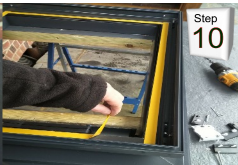
Peel off the protective paper on glazing seals.
