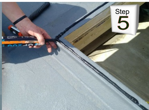
Lay an even bed of sealant around the upstand.
