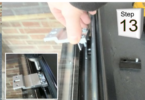
Screw motor arm back onto lid.
