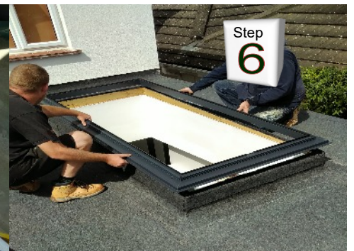
With the lid removed (see front page) bed down frame.
