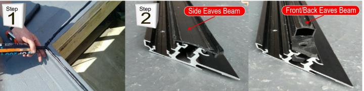
Lay down an even bed of silicone on the prepared upstand.
