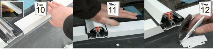
Peel back tape, position trim equally Clip down top caps all the way between rafters, tape side to glass.
