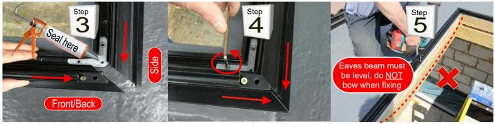
Use ratchet cleats to join eaves beam mitres. Seal mitres first.
