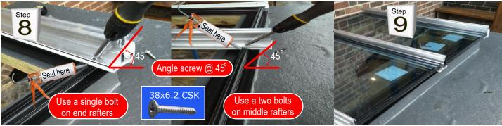
Screw rafters to eaves beam. Position screws at a 45 degree angle to locate into eaves beam (as shown).
