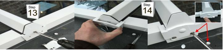
Only use middle hole (as shown). Fit plastic cover plate on to the aluminium end plate using two screws to the lower holes. Fit screw cover caps.
