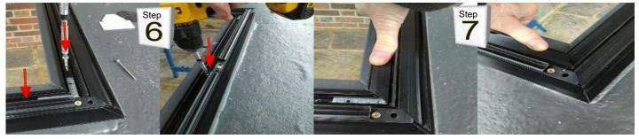
Drill a 5mm pilot hole at fixing point. Fix either side of mitre cleat and behind each middle rafter point.
