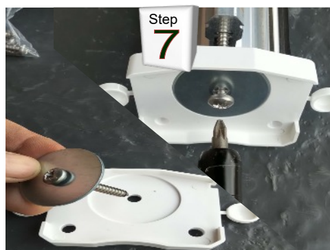
Fix glass retainers on ends of the rafters
