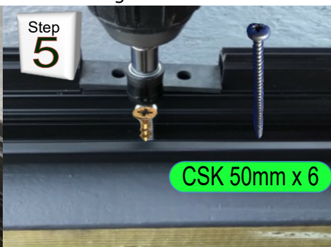
Fix eaves beam to your upstand with screws provided
