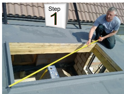
Check opening is square and level.
