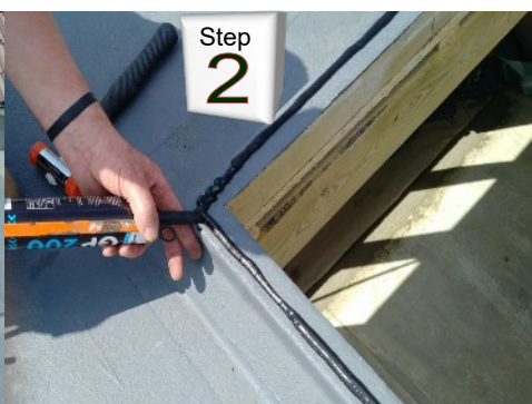
Seal top of up-stand before fitting eaves beam.
