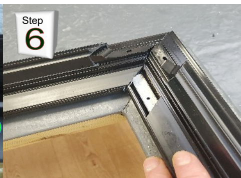
Clip on internal screw cover trim.
