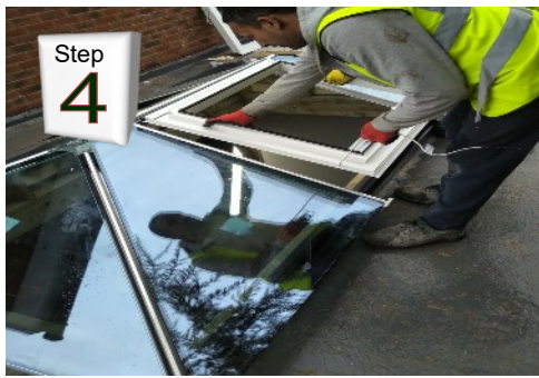
With the lid removed fit the vent into roof opening
