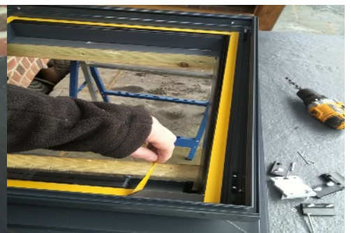
Peel off the protective paper on glazing seals
