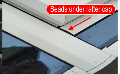
When roof top caps go on make sure beads fit under caps
