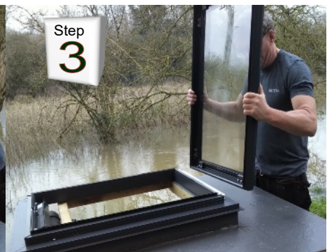
Disengage the opening catch from the vent lid. Open lid to 45 degree then lid will come away from the vent frame
