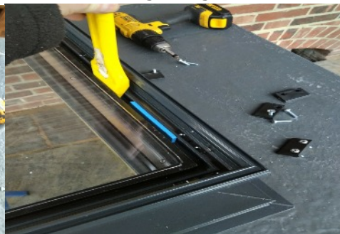
Pack glass unit evenly with glazing packers
