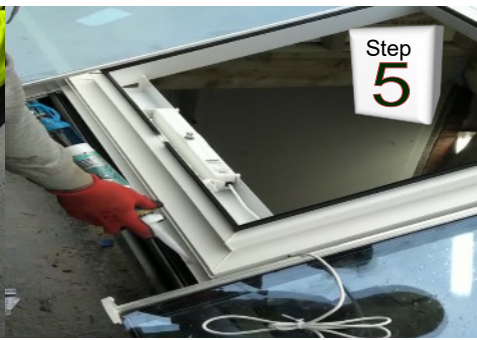
Before glazing the lower panel lay a bed of neutral cure sealant
