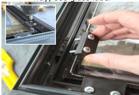
Clamp glass with clamp blocks, these fit to travellers in frame
