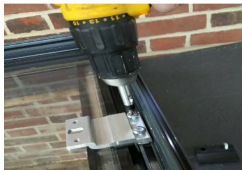
Remove motor arm from lid prior to glazing
