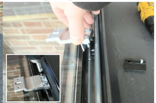
Screw motor arm back onto lid
