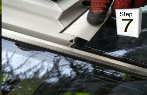
Clip cover bead into channel
