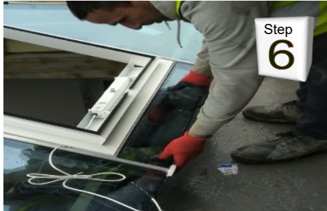
Glaze lower panel making sure there is a good seal to vent
