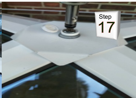
Screw down top cap plate
