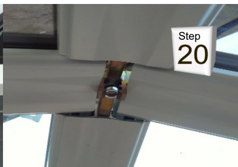
Make sure nut is in radius end before fitting cover plate
