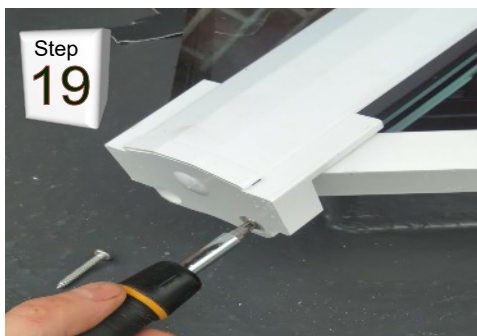
Screw and clip on screw covers
