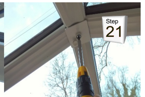
Finally screw on internal cover plate
