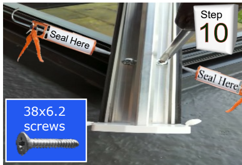
Seal then secure rafter into eaves beam with 38x6.2 screws
