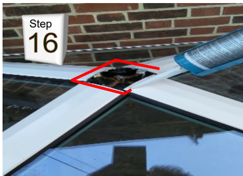
Seal around top before fitting cap plate
