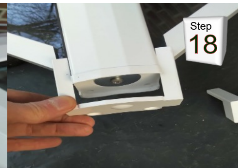
Fix rafter face plates
