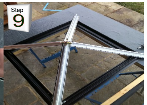
Lower all the rafters on to eaves beam
