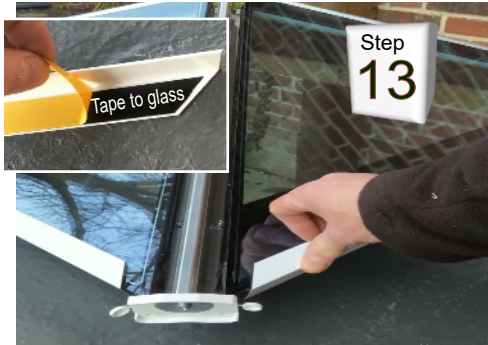
Peel off glass closer backing and position between rafters
