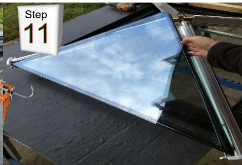
Fit glass units facing correct way (see glass label)
