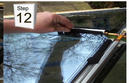
Push draft foam at the top of each rafter
