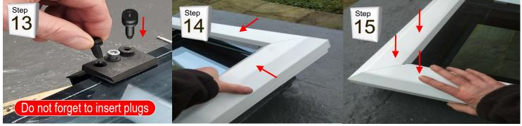
Insert x2 rubber plugs, one either side of the bolt as shown.
