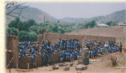
Schul-Baustelle in Banyo 2014
