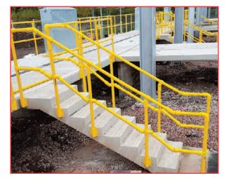
Tubular handrail system is particularly simple to install on site. The tube can be cut to size and matching pairs of moulded fittings can be fixed to the tube to complete the system.
