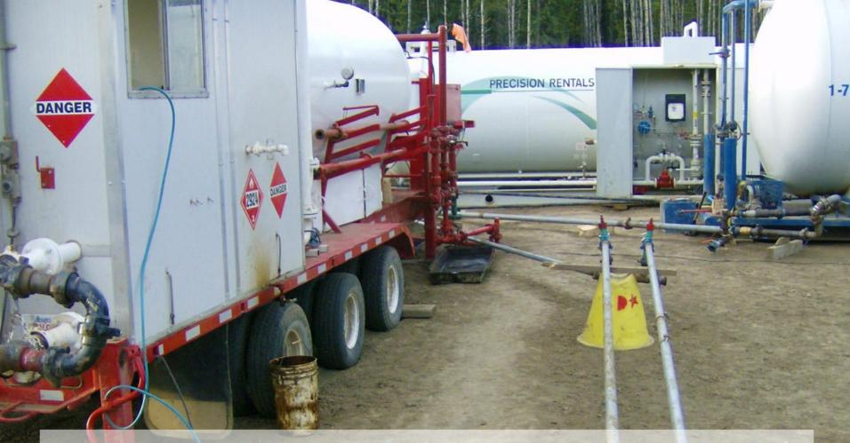
The Vented flash off from the propane holding tankers are recapture intentionally designed to be recirclate back upstream of heat exchanger for processing the vented flash off
