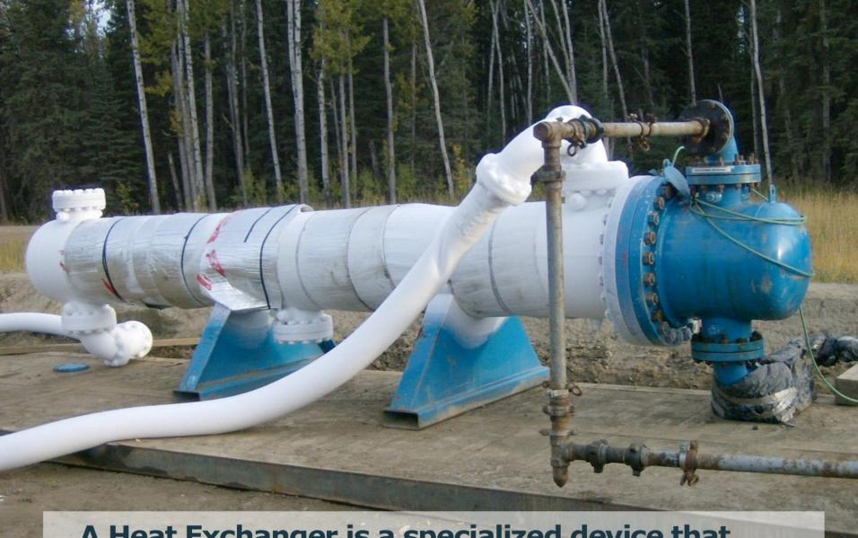
A Heat Exchanger is a specialized device that assists transfer of heat from one fluid to the other
