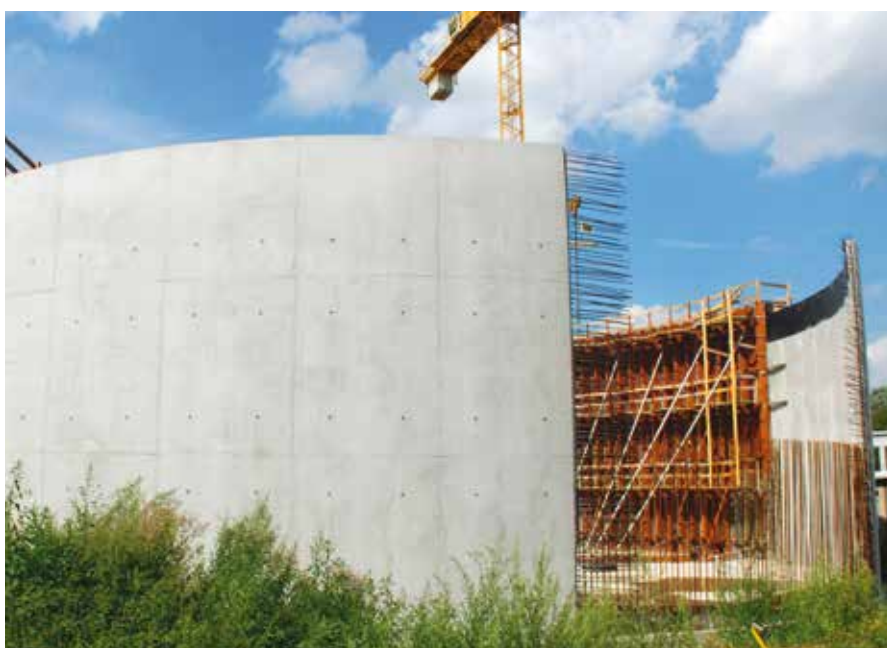
Biogasanlage, Bürstadt; Fa. Wilms, Bürstadt
