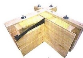
Single log wall with additional insulation
