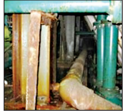
Equipment Corrosion of Traditional Wet Bottom Ash Handling System.
