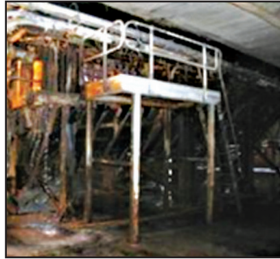
Equipment Corrosion of Traditional Wet Bottom Ash Handling System.
