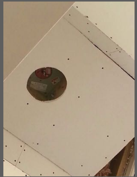
Winch fitted below the ceiling and concealed within the ceiling rose
