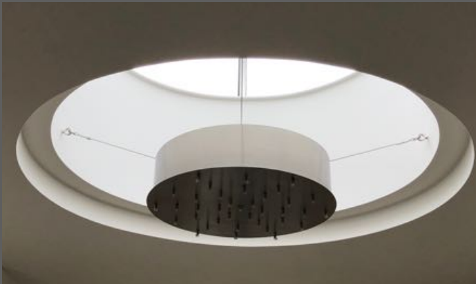
Winch concealed within the ceiling rose and side suspended
